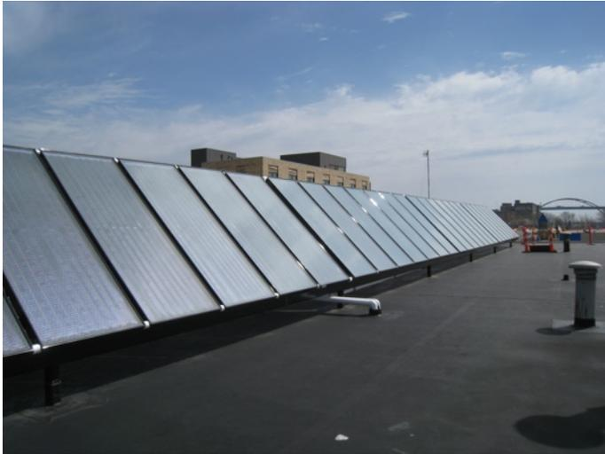
project will reduce the brewery's energy costs as well as showcase the company's commitment to sustainable brewing practices. The installation includes 28 solar panels located on the roof, which will be used to pre-heat the water used in the brewing process.
